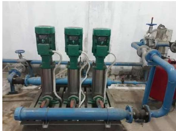
Gambar 4.1 Multiple Pompa Booster
