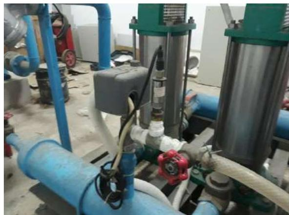
Gambar 4.2 Sensor / Switch Pressure
